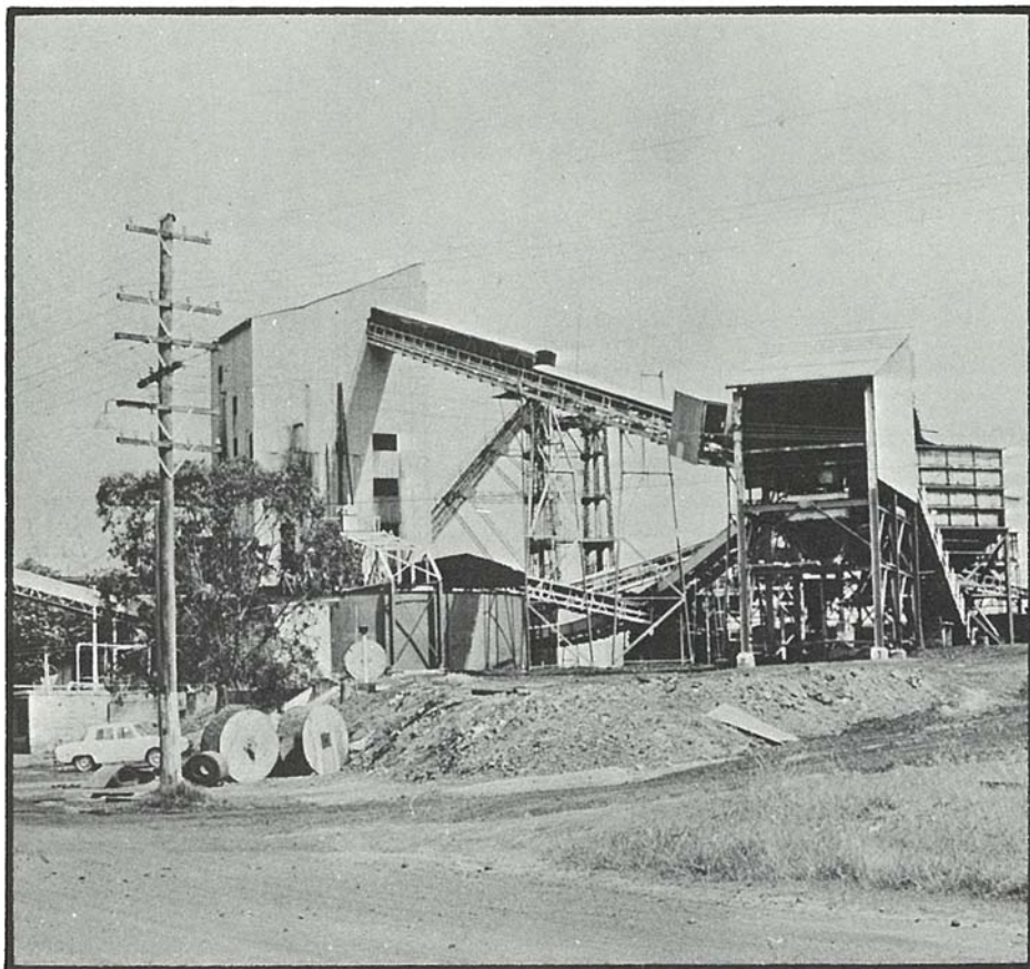
A coal washery near Newcastle.
