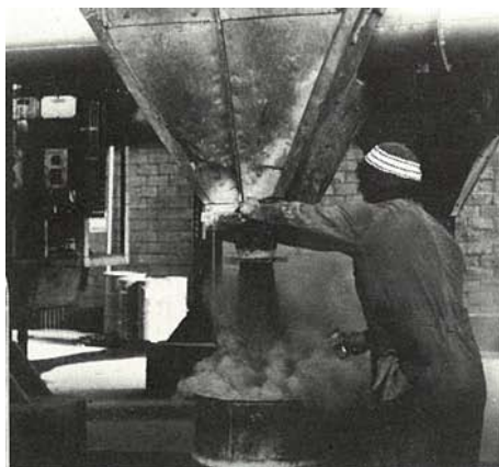
Fly-ash being emptied from an electrostatic precipitator.
