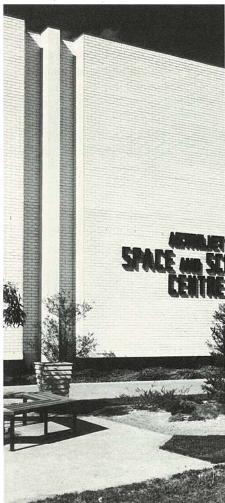
The white-surfaced engobed bricks in this building at Melbourne airport contain crushed waste glass.
