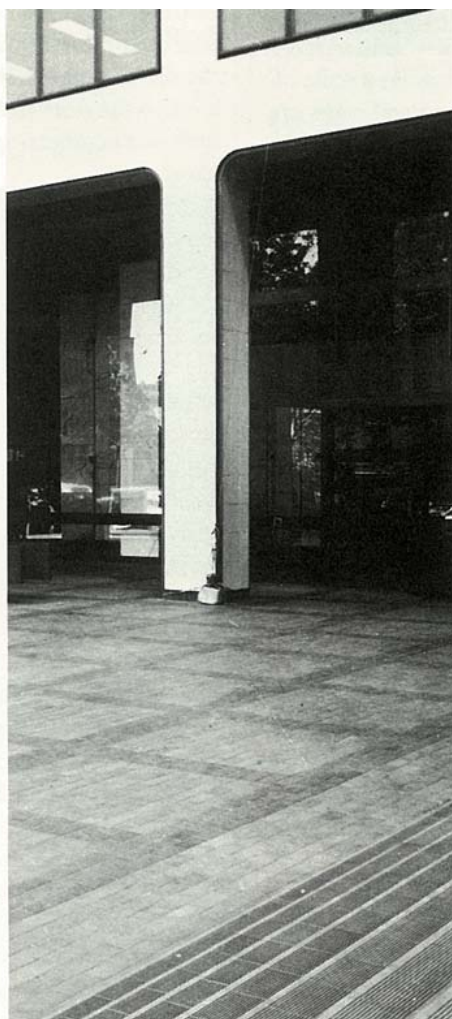
Tiles made from basalt dust pave the forecourt outside this Melbourne building.
