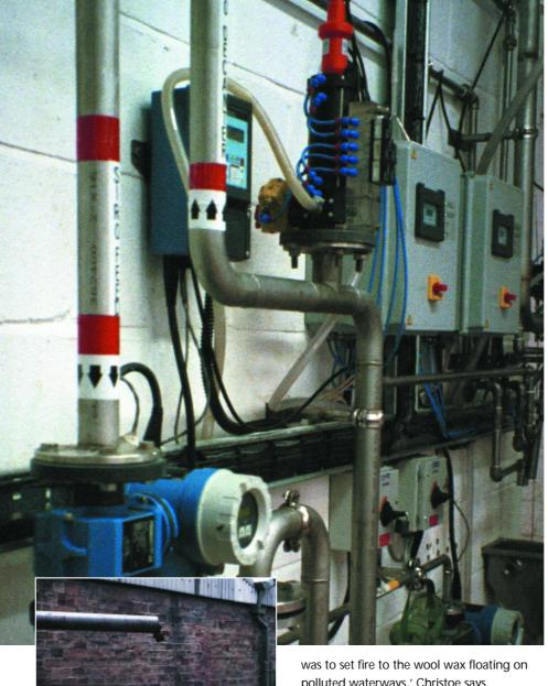
The Sirolan SWIMS system separates wastewater into three streams, enabling wool mills to optimise the removal of scour contaminants before discharge to effluent treatment systems. The resulting sludge from dirt and wool wax meets all the requirements for a high grade potting mix or broadacre soil conditioner.
