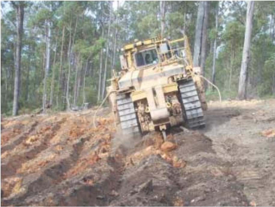
A disused mine pit is ripped to a depth of 1.5 metres in preparation for seed application by an air-seeder mounted on a bulldozer. Deep-ripping breaks up the compacted ground and the ripping mounds prevent soil erosion.
