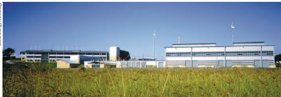
The new National Energy Centre in Newcastle is a working demonstration of the latest renewable energy technologies.
