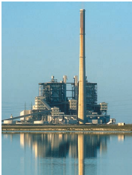
A power station at the head of Spencer Gulf, SA, where brown coal from Leigh Creek South is used to generate electricity.
