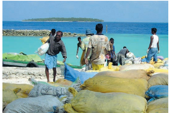
Maldivians unload reconstruction material to repair tsunami-damaged buildings. The Maldives sit just a metre above sea level in the Indian Ocean, south-west of Sri Lanka. CSIRO Marine Research
