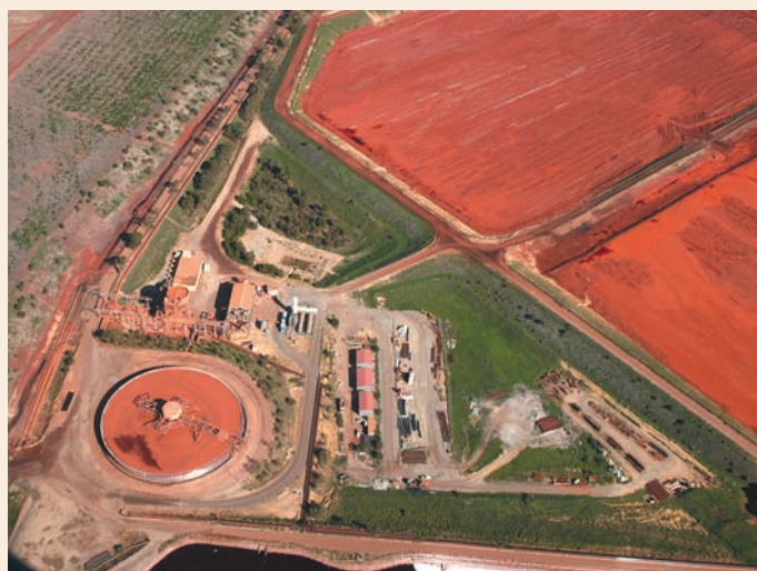
The Kwinana refinery's mud residue carbonation facility. Alcoa
