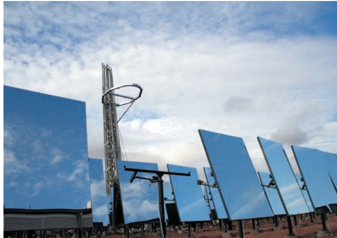
The mirror array of the solar reactor at CSIRO's Energy Technology Centre, Newcastle. Nick Pittas
