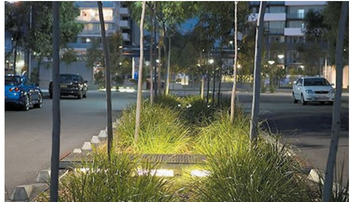
The new native rain gardens are aesthetic collection and filtration points for stormwater. Tony Wong/FAWB
