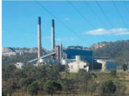
The Callide A power station near Biloela will advance confidence in oxy-fuel technology.
