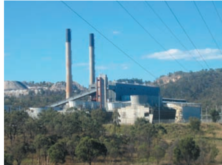
The Callide A power station near Biloela will advance confidence in oxy-fuel technology.
