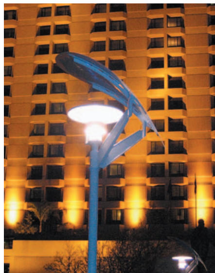
Solar lighting in Victoria Square, Adelaide.
