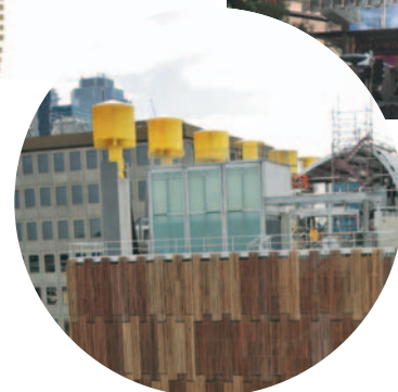
The City of Melbourne’s new Head Office, CH2, is one of only a few 6 Star Green Star–Office Design rated buildings in the world, and features external wooden louvres (far right) and wind-powered extraction vents on the roof (right). Green Building Council of Australia
