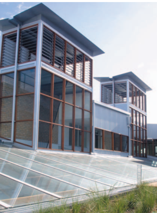
Melbourne's pace-setting 60L building has thermal chimneys, a glazed atrium roof and a rooftop garden as energy efficiency measures, among an impressive list of other innovations that are attracting clients. Dare images, courtesy The Green Building Partnership
