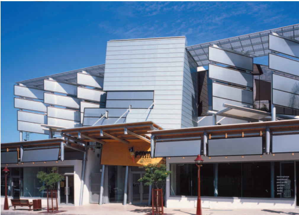
743 Ann Street, Brisbane, had a sustainability upgrade and includes an external thermosiphon ventilation system. Green Building Council of Australia
