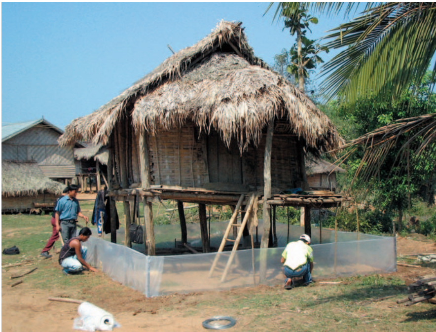
A barrier of plastic sheeting is erected around a village grain store. Holes in the plastic lead to traps inside the barrier. CSIRO
