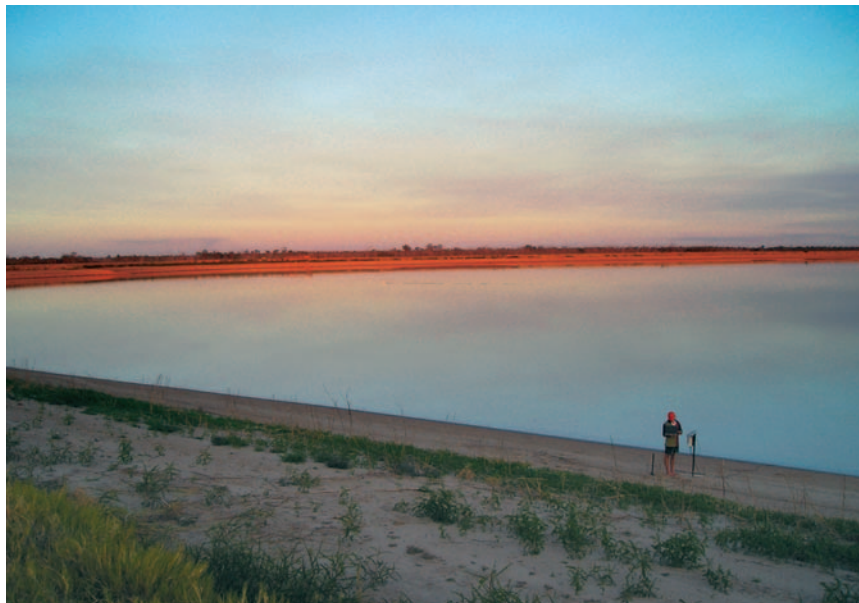
While plastic covers can be used to prevent evaporation from small dams, spray or pump-on monolayers are more appropriate for large dams like this one. CRC for Irrigation Futures
