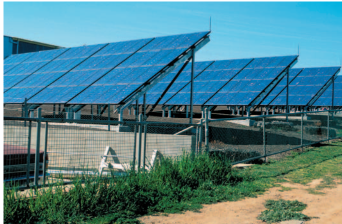
Solar panels at Queanbean, NSW. Renewable energy featured in COAG's decision-making on energy supply and climate change impacts. Greg Heath/CSIRO
