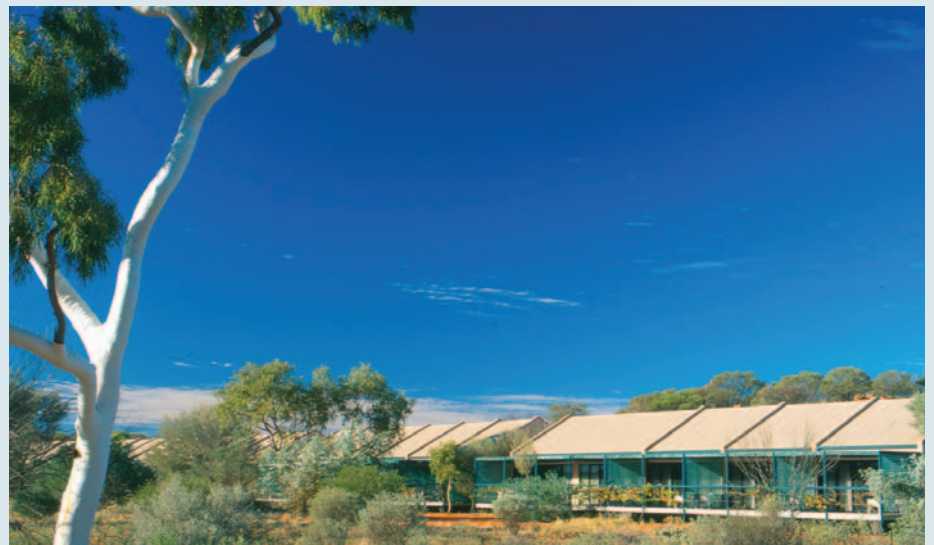
Voyages' Kings Canyon Resort runs partially on solar power and recycled groundwater. Voyages
