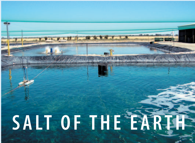
The innovative research and demonstration facility at the Inland Saline Aquaculture Research Centre, Wakool. ISARC
