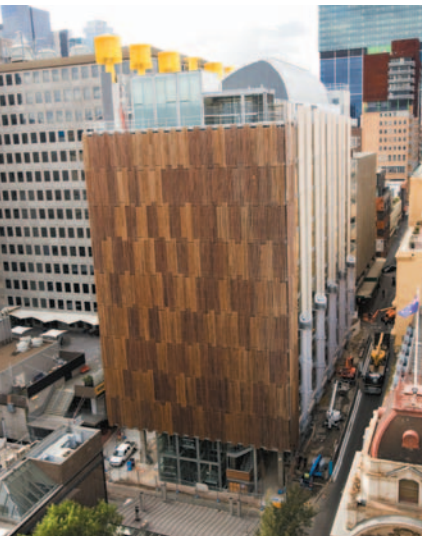
A focus on high-rise buildings' environmental efficiency is spurring rapid advances in design technology, such as that seen in Melbourne's CH2 building. Melbourne City Council
