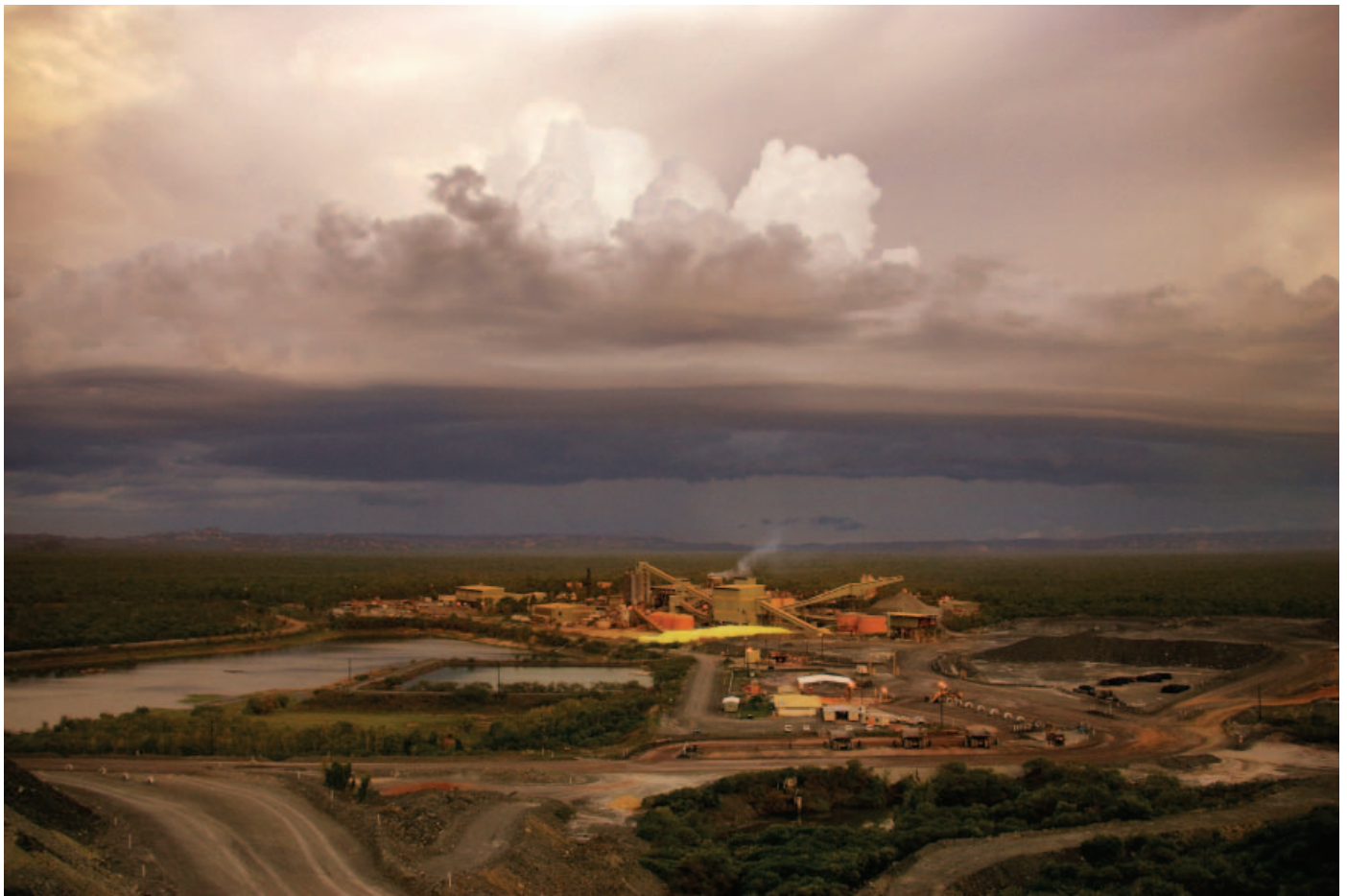
ERA's Ranger mine site in the Northern Territory, in the midst of the undeveloped Jabiluka uranium deposit. ERA
