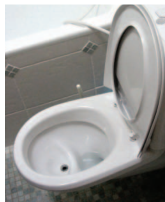
A trial of urine-separation toilets is currently underway in Queensland.
