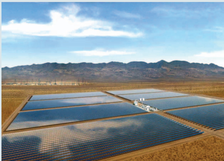
The US has been forging ahead with solar thermal power. Acciona's Nevada Solar One™, an enormous solar thermal concentrator array, can generate 64 megawatts – enough to power 14,000 households. Acciona
