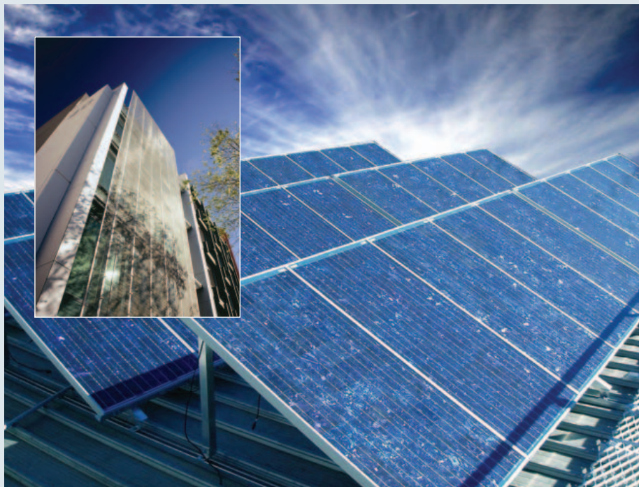
Energy efficient building design can dramatically reduce energy consumption – the Szencorp office building in Melbourne has a 6-star rating and includes its own photovoltaic energy supply on the roof. Szencorp
