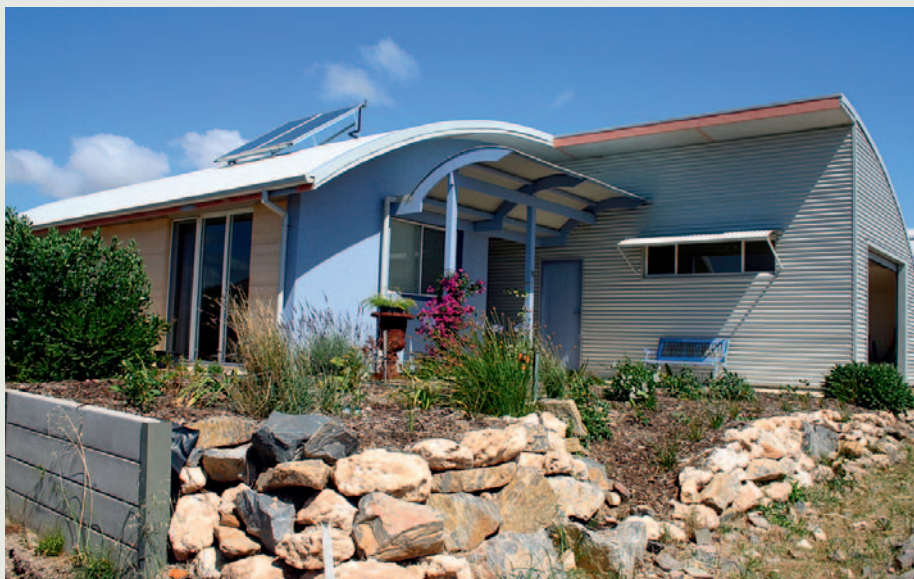
Ecovillages are characterised by sustainably designed homes with northerly orientation for passive solar heating, eaves, solar hot water, rainwater tanks and other sustainable living features. Vanda Rounsefell
