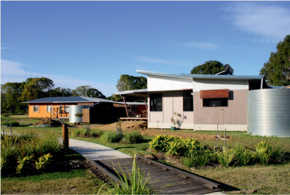
The EcoVillage at Currumbin, Queensland, is designed to make it easier to cycle or walk to the Village Centre rather than use a car, with all facilities located within walking distance of every home. Currumbin EcoVillage
