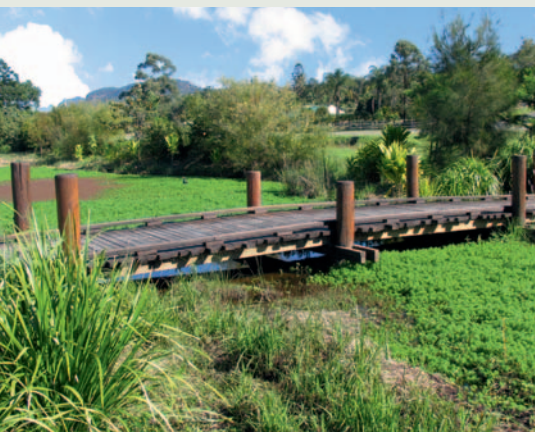
Stormwater at The Ecovillage, Currumbin, is kept in the environment via swales to maintain landscape features such as ponds.
