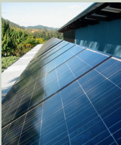
Photovoltaic array on the roof of the community EcoCentre at Crystal Waters Permaculture Village. Excess solar energy is sold to the grid. EcoLogical Solutions
