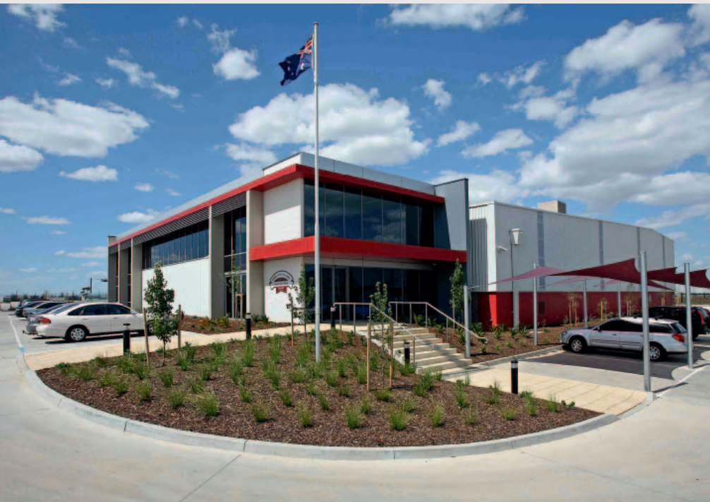
Left: Ferguson Plarre’s new bakehouse in Melbourne includes hot water generation using heat reclaimed from refrigeration, monitoring of energy and water consumption, and rainwater tanks for toilet flushing, irrigation and truck washing. Ferguson Plarre
