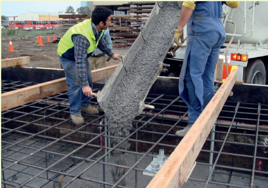
E-Crete uses waste fly ash and slag to achieve a comparable cement for an 80 per cent emissions reduction. AP/Zeobond
