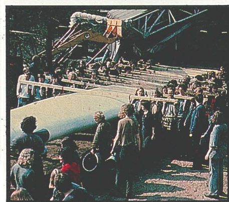
Volunteers roll one of the blades of the Tvindmill out of the hangar where it was constructed.
