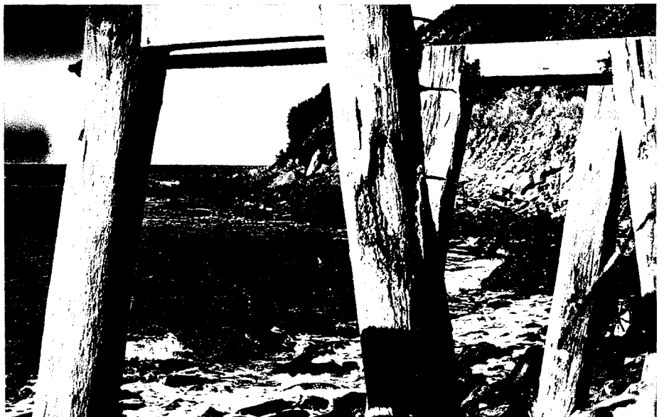
All that remains of the sea wall that was built in 1949 at Clarke's Slip a few kilometres east of Lorne, Vic., to protect the Great Ocean Road. Rock fill was stacked as high as the top of the piles.
