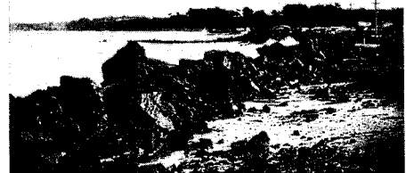
Not even basalt sea walls prevent erosion of the beaches round Portland Bay. Here the sea has eaten out the dune behind the wall.
