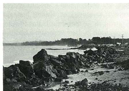
Not even basalt sea walls prevent erosion of the beaches round Portland Bay. Here the sea has eaten out the dune behind the wall.
