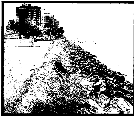
Rocks forming a sea wall at Surfers Paradise have proved no substitute for the original foredunes.
