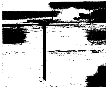
Henty Bay Estate, east of Portland, Vic. These pipes once lined bores for pumping up fresh water onto blocks of land located along the shoreline.
