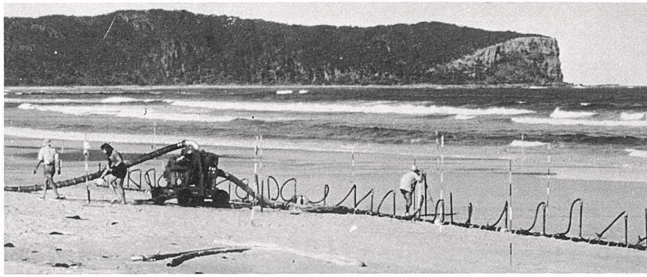
Staff and students from the Geography Department of the Australian National University study how pumping water out of the beach increases sand deposition at Durras Beach, N.S.W.
