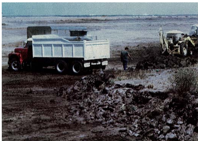
Harvesting sewerage sludge from the drying lagoons at Bolivar, S.A.
