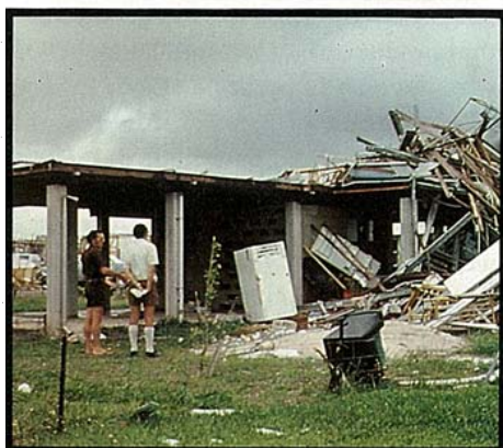
Two houses on stilts — severe racking distortion (above) and total demolition (below) above floor level.
