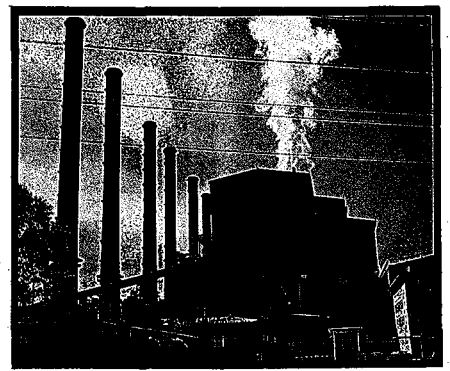
Hazelwood power station, in the LaTrobe Valley, Victoria, burns brown coal to help meet the base load.
