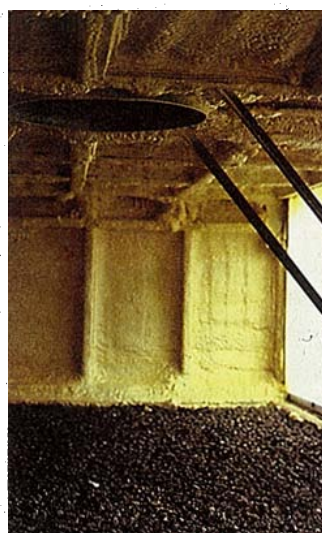
The rock pile and fan. The outer walls are insulated to reduce heat loss.
