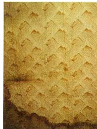
The 'tide mark' rises up a damp wall.
