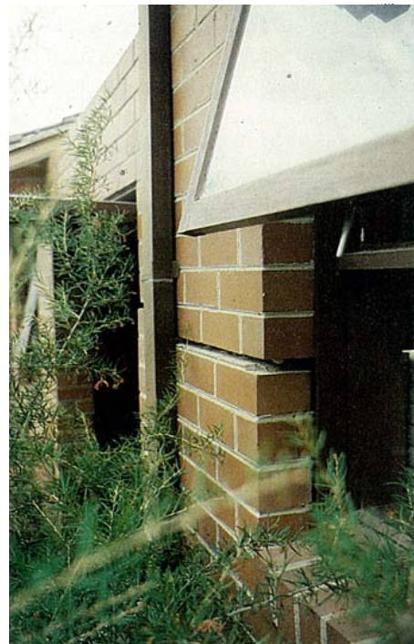
A 'tree-damaged' building in the Melbourne suburb of Ringwood. Soil drying has produced shrinkage settlement of the footing.
