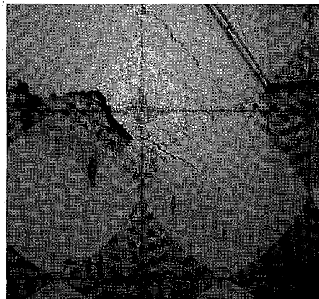
Trees near the South Australian Art Gallery dried out the soil, cracking the Gallery wall. Things improved after the trees were removed.
