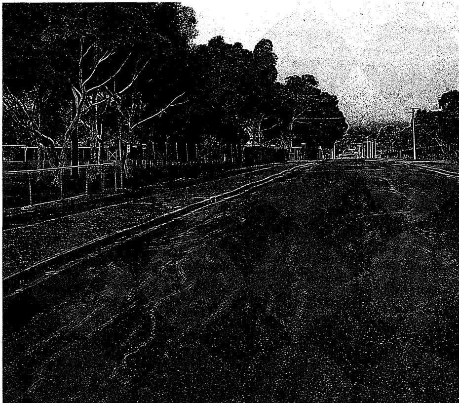
A cracked road in Adelaide. The soil beneath it is a black earth.
