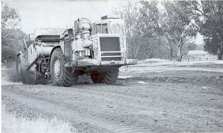
... and mixing it into sandy soil using an earthmoving 'scraper'.
