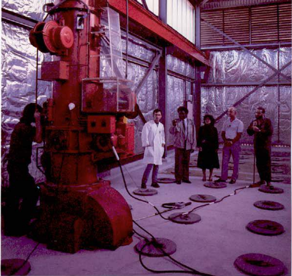
At Lucas Heights, spent fuel elements are held in stainless-steel-lined holes 16 m deep. Inspectors from the International Atomic Energy Agency are checking that all is well.
