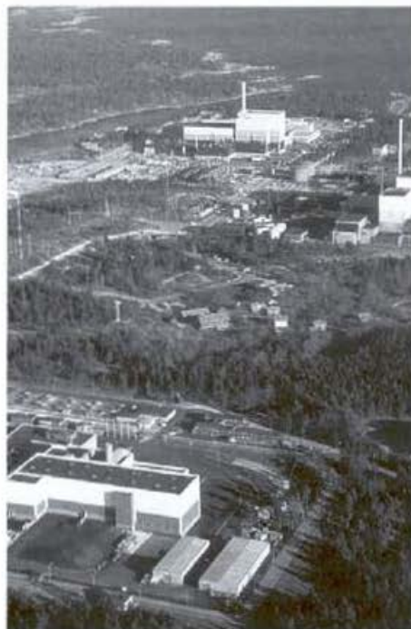
The Oskarshamn nuclear complex in Sweden. Three power plants are in the background; in the foreground are the surface buildings of the Central Facility for Intermediate Storage of Spent Fuel (CLAB).
