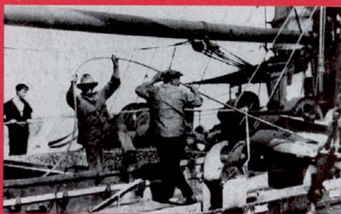
Laying cable earlier this century.
