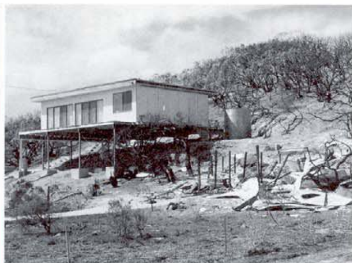
What could have saved this one?
