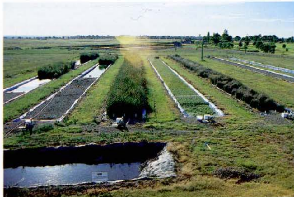
The experimental trenches at the University of Western Sydney, designed to receive some 400 000 litres of effluent per day.
