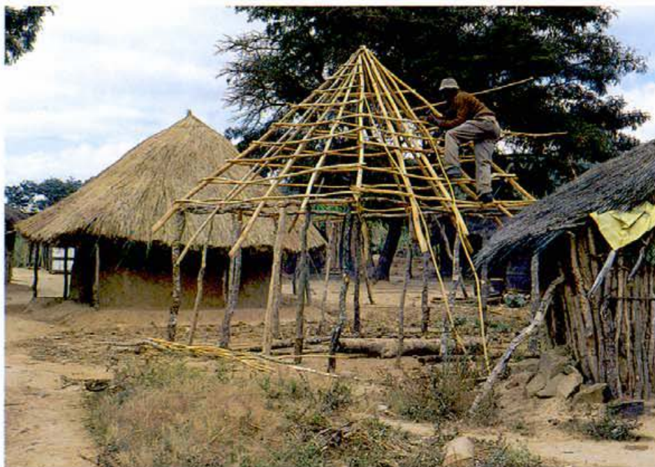
Poles from fast-growing young eucalypts make low-cost, durable construction material.
