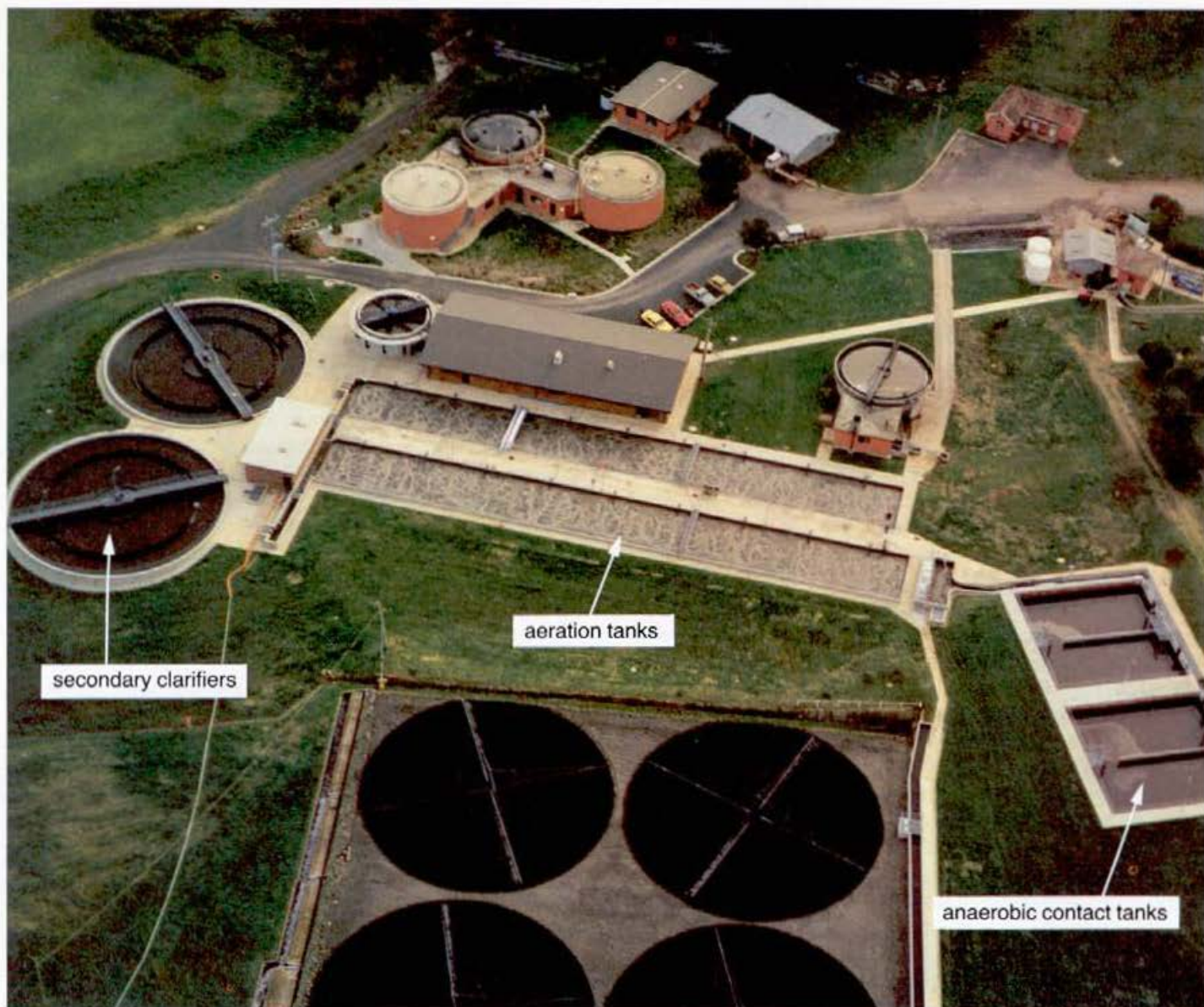
The full-scale biological phosphorus-removal plant designed by CSIRO stretches across the centre of the picture. The main elements are labelled.
