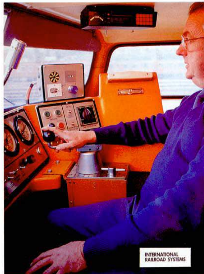
Metromiser in the train cabin.
