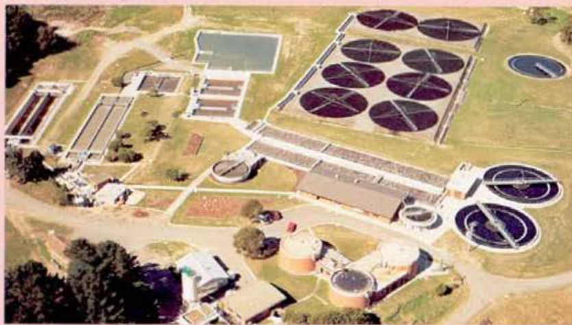
Ballarat South waste-water treatment plant.
