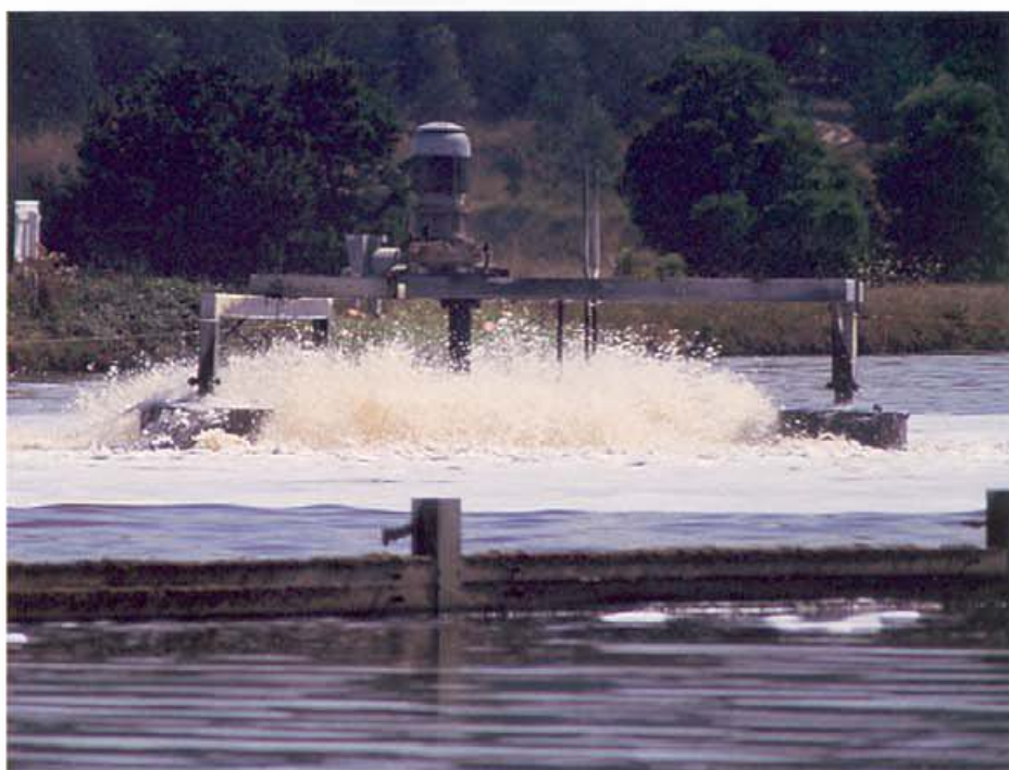
Effluent discharge from the Australian Paper Mills plant in Gippsland is treated through a series of aerobic and anaerobic ponds.
