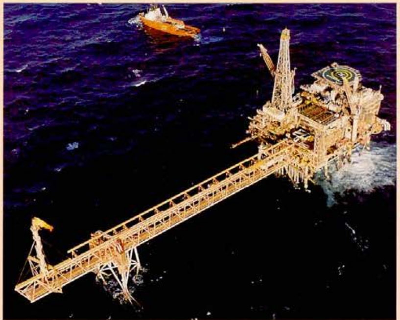
Woodside Petroleum's North Rankin gas production platform: designed to safely withstand the '100-year return period storm'.
