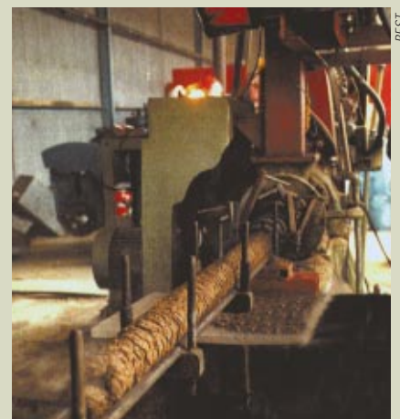
A range of biomass fuel sources will be briquetted at the demonstration plant.
