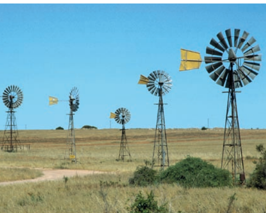
A cluster of windmills pumping groundwater at Penong, SA. Willem van Aken, CSIRO
