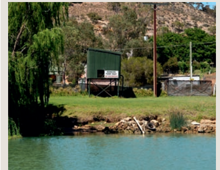
A domestic pump on the banks of the River Murray at Younghusband, SA.
